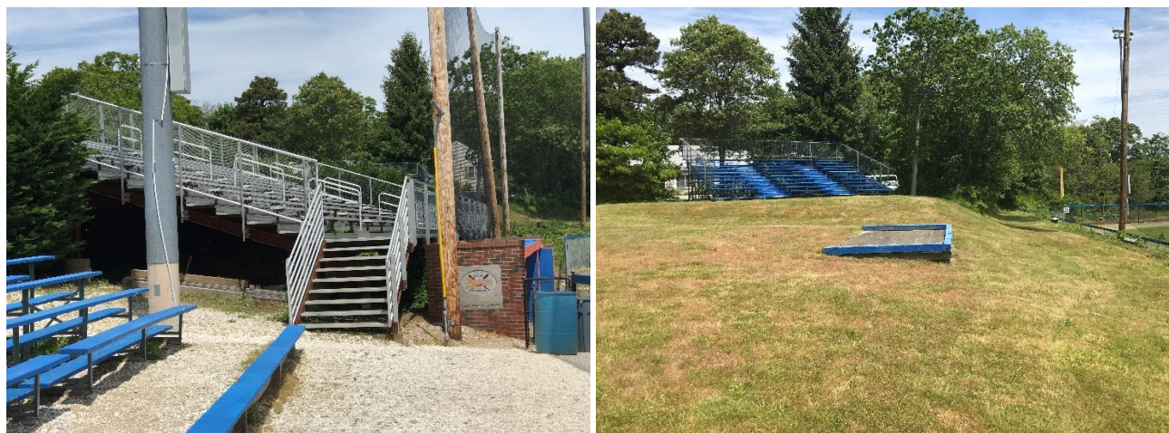
Mckeon Field lacks accessible routes to any of the field amenities, including bleachers, concessions building, or the field.
