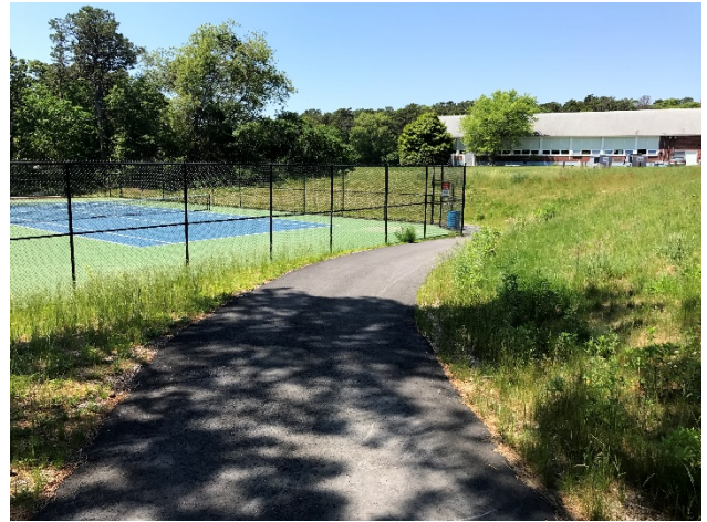
Accessible Route to Courts, Barnstable West Barnstable Elementary
