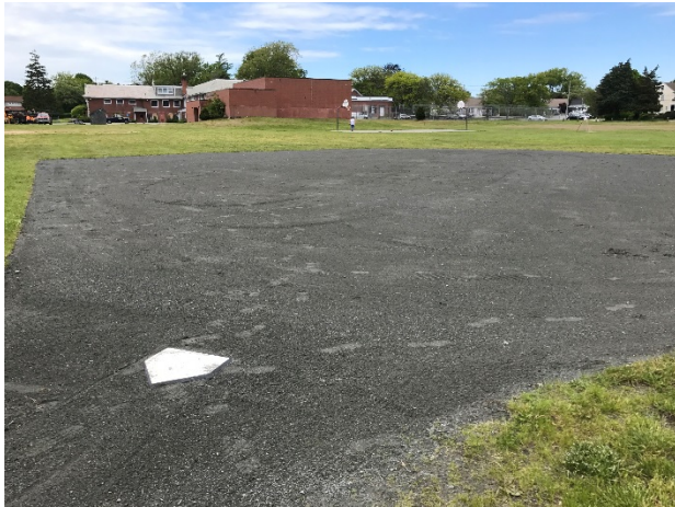
Stone dust Infield, Osterville Bay Elementary School
